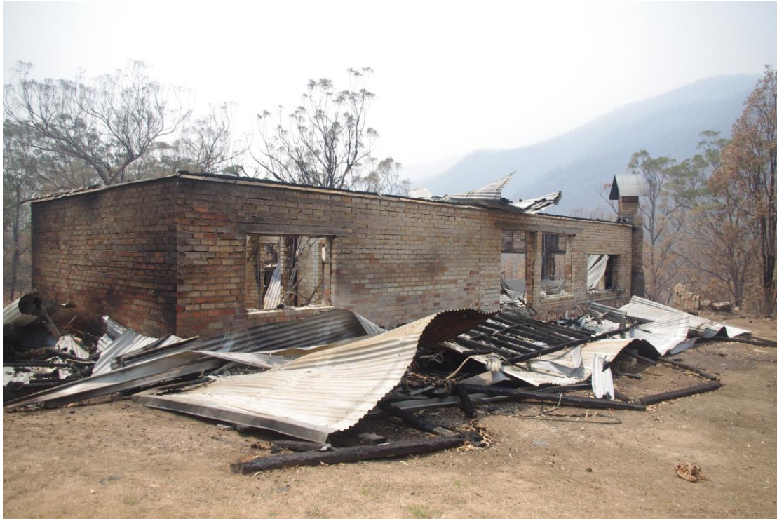
This house on the South West corner of Wyalaliba was destroyed just before completion.
